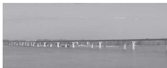
Figure 10. Volgograd bridge. A multi span continuous girder motorway bridge spanning 120 m - 150 m between piers.
