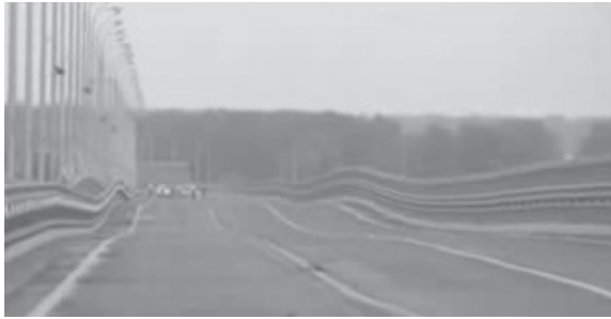
Figure 11. YouTube video clip taken along the Volgograd bridge displaying vertical oscillations.
